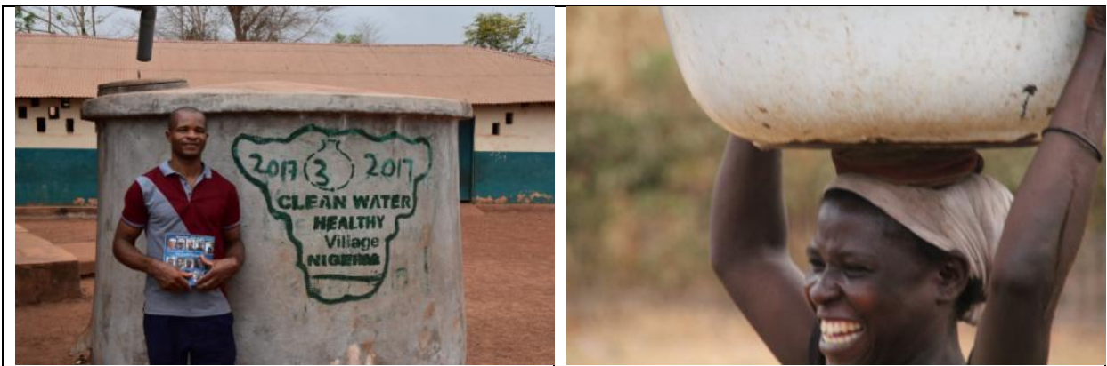
Water project, in Nwofe Agbaja. The Izzi people are very enthusiastic about the construction of water tanks (left) to provide drinking water in the dry season (right). The concept is taken from Guinea-Bissau and introduced in Nigeria in 2017-2018. Construction teams will be inclusive.
